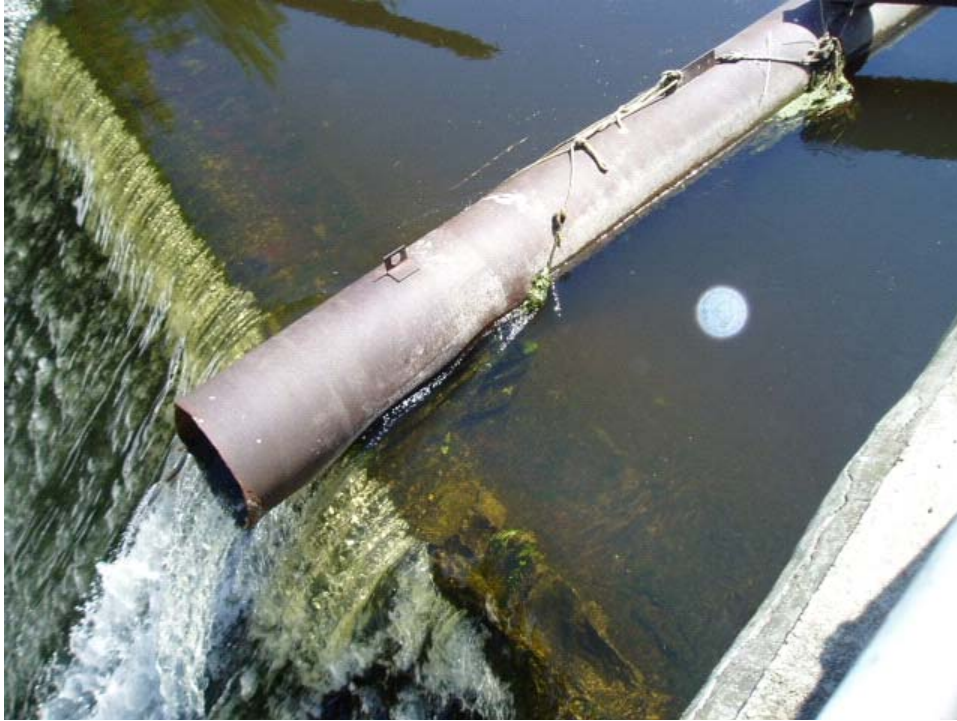
Photo 4. Spillway of Columbia Mill Dam with mill process water effluent pipe.
