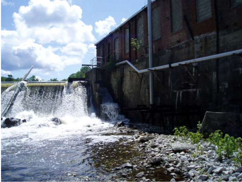
Photo 7. Upstream view of Columbia Mill and Columbia Mill Dam.
