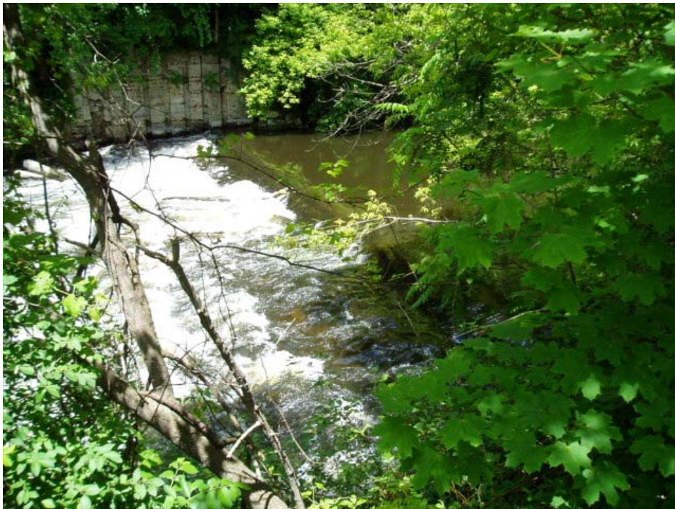
Photo 12. View of Eagle Mill Dam remnants from left bank.
