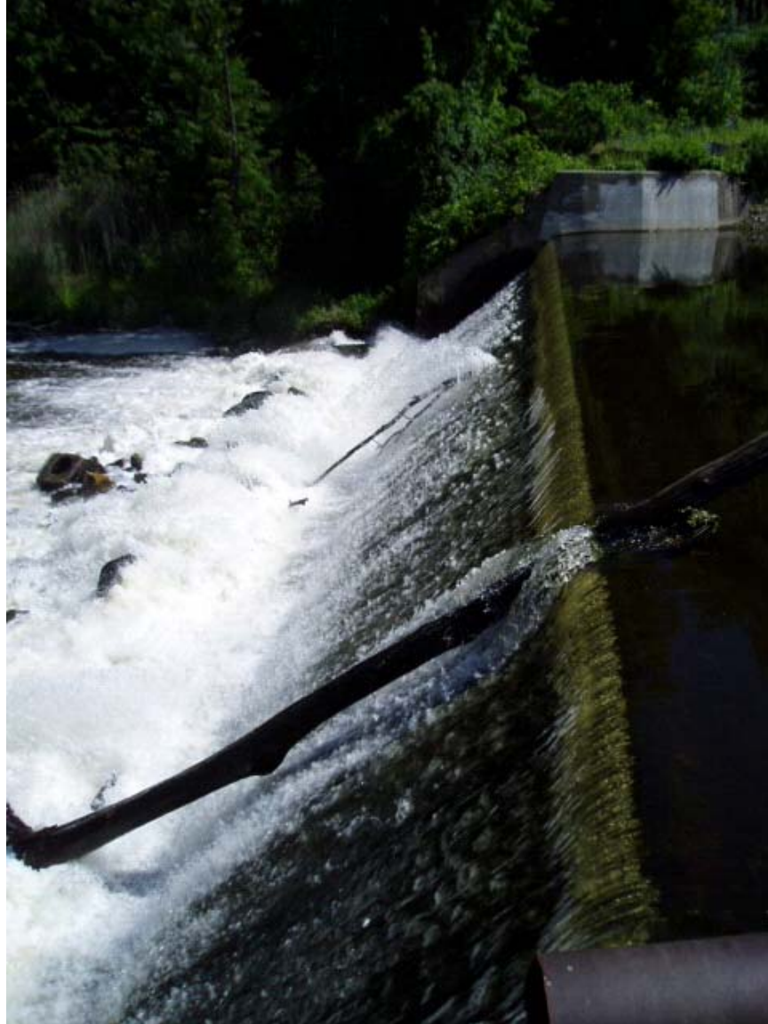
Photo 1. Columbia Mill Dam from left bank with woody debris.
