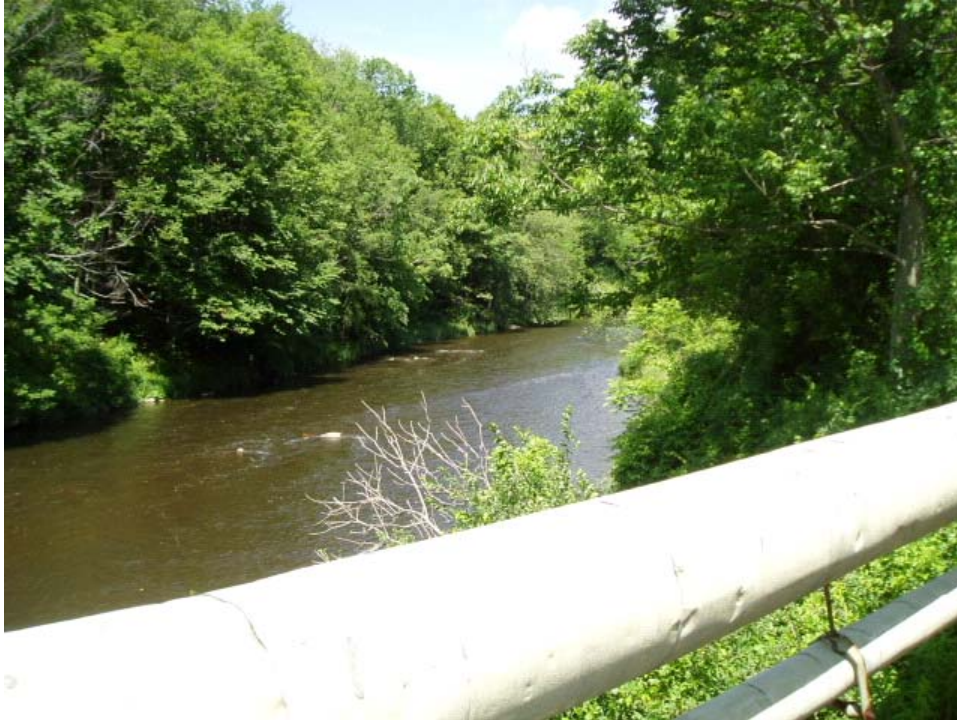
Photo 11. View of in-stream pipe alignment below Columbia Mill Dam (straight line in water). Note that pipe in foreground is currently undergoing removal.
