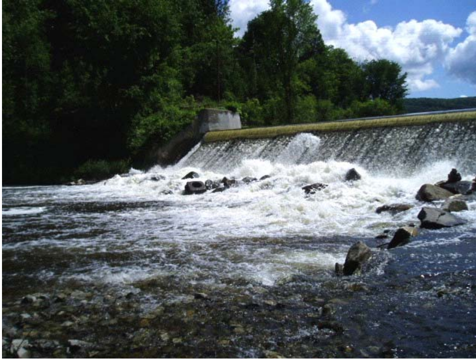
Photo 2. Upstream view of Columbia Mill Dam.
