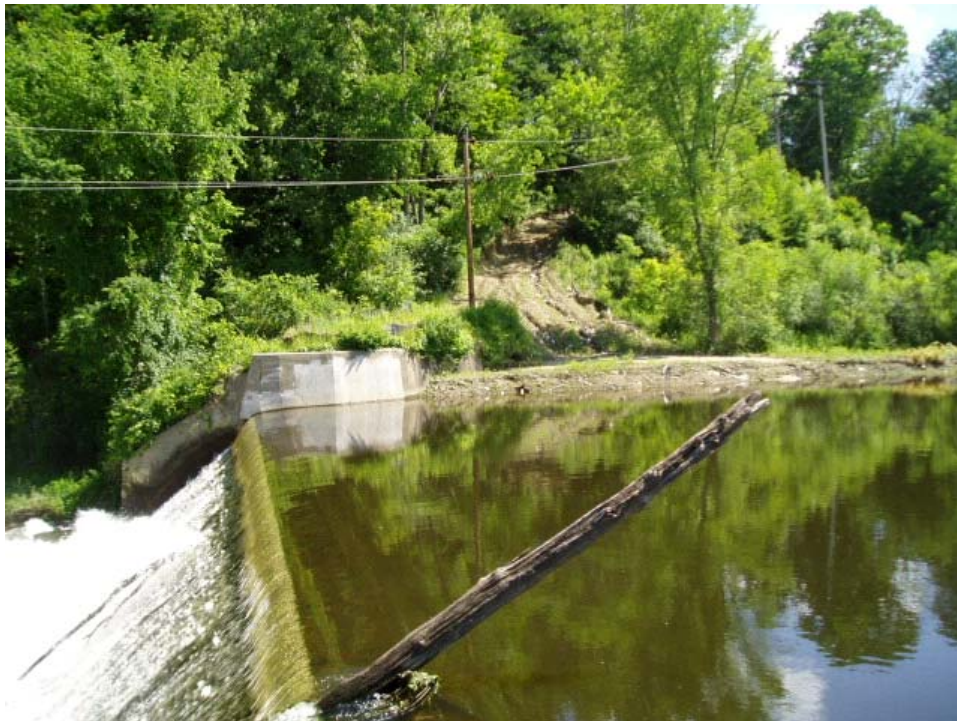
Photo 3. Columbia Mill Dam from left bank showing potential construction access road.
