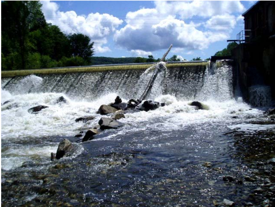
Photo 5. Upstream view of Columbia Mill Dam.
